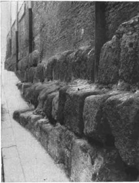
Fig. 96a. S. Martino ai Monti, Ninth century basilica, foundation and rising wall of east aisle
